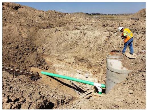
• NRE has installed the outside drop main connection to sanitary sewer manhole 11.
