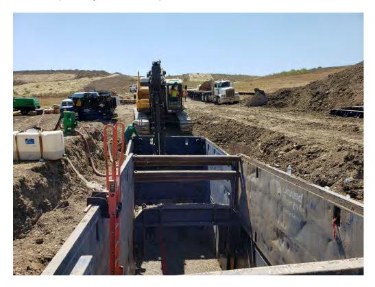
NRE has completed the bore below Big Dry Creek. Installation of fusible carrier pipe is pending material delivery. NRE to run carrier pipe through Jefferson Parkway ROW casing, Big Dry Creek casing and connect to existing stub at Noble St.
