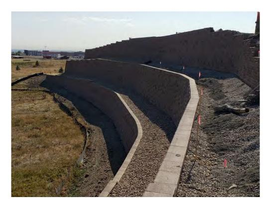
• The phase 1 retaining wall block is complete with cap. Rock mulch between tiers and blanket on the bottom slope are yet to be completed.
