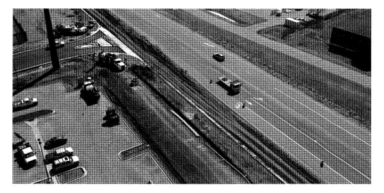
Bottom lift paving is done on Yankee Street and West 92<sup>nd</sup> Drive to the east side of the Xcel substation. Paving for the Highway 72 widening is scheduled for the end of this week.
