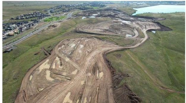
Phase 2 Facing East
