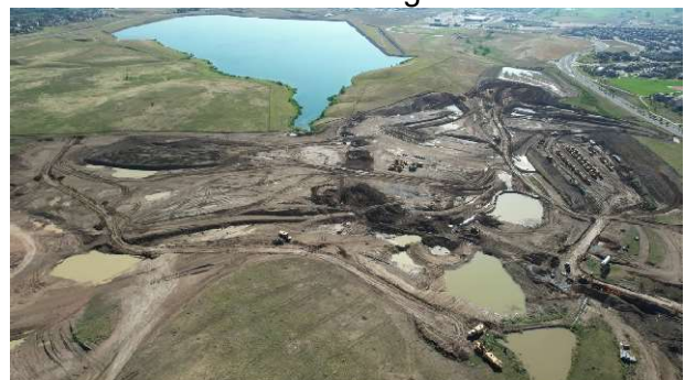
Phase 1 Facing South
