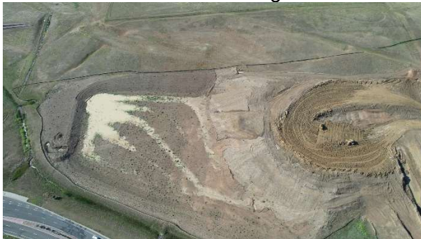
Future Detention Pond
