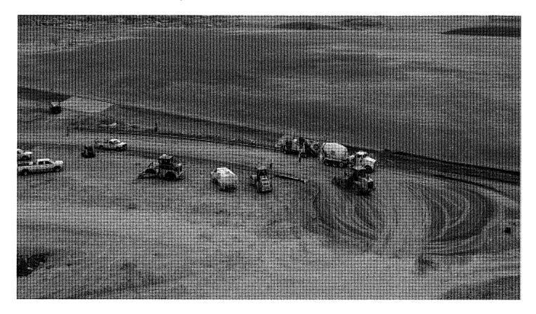
• Kelley Trucking is cutting the stockpile and moving material to the west side of the project.
