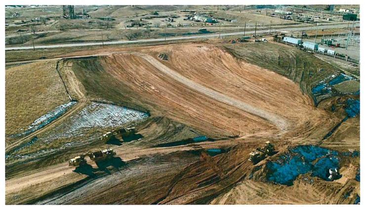
Grading and structures for the drainage pond are complete and storm pipe going to the pond is installed.
