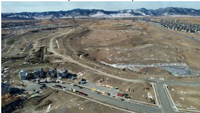
Block 13 Overview (View: West)
