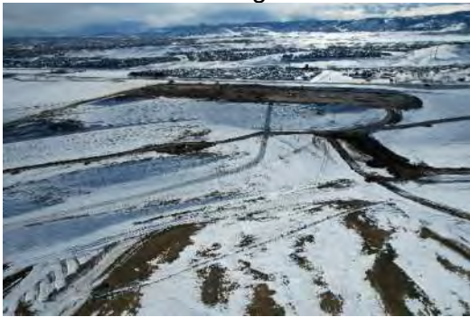
Phase 2 facing North
