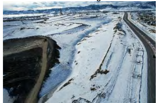
Phase 1A Facing Southeast
