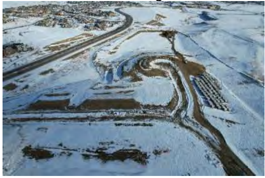
Phase 1A Aerial facing East
