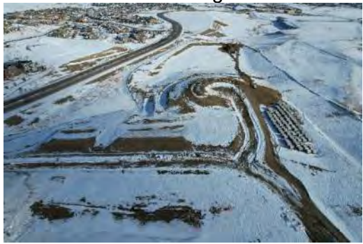
Phase 1A Aerial facing East
