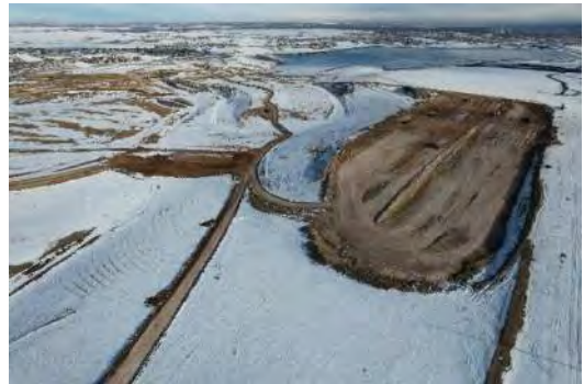
Phase 1B facing Northwest
