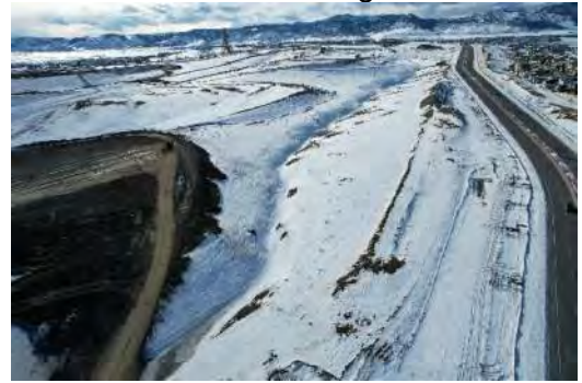
Phase 1A Facing Southeast
