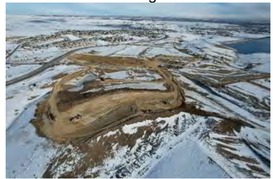
Phase 1A facing Northeast
