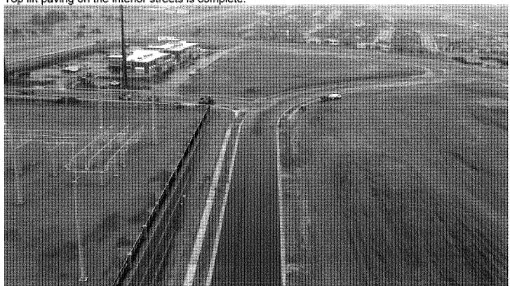
Bottom lift paving is installed for 80% of the Highway 72 widening. The remaining bottom lift
