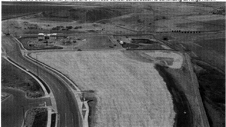
The pond grading was revised to meet the required volume and outflow for certification by Galloway. The riprap at the inlet to the pond was rebuilt per comments by the city.
