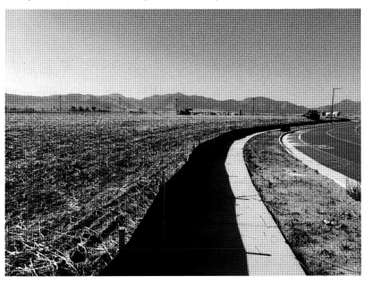
PEI has constructed the revised maintenance access road and swale in the detention pond to alleviate drainage issues. The overflow spillway was regraded to a defined channel and Turf Reinforcement Mat was installed.
