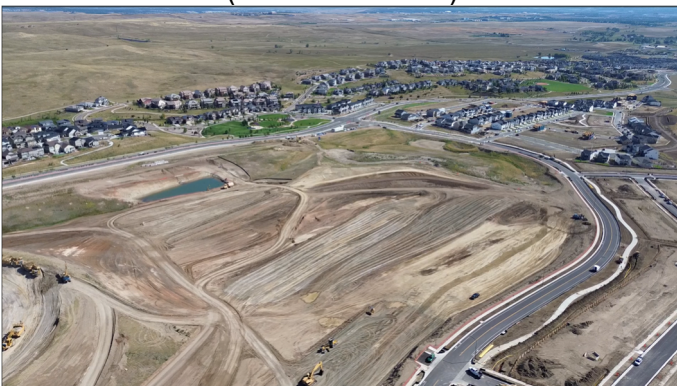
Trailstone Grading (View: Northeast)
